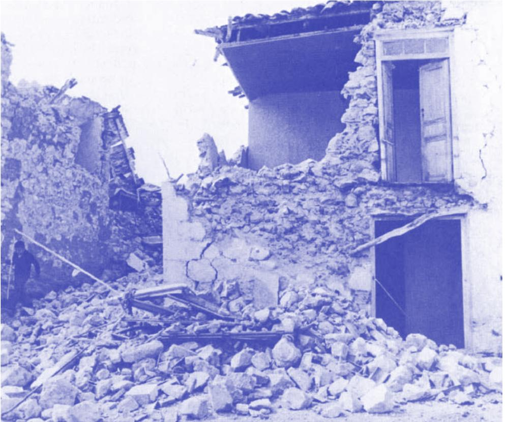
This masonry house in Corinth, Greece was badly damaged in the earthquake of March 1981. Inadequate bracking of stones, and the use of mud mortar were two reasons for the failure. Techniques can be communicated to local craftsmen on a seismic building techniques.
