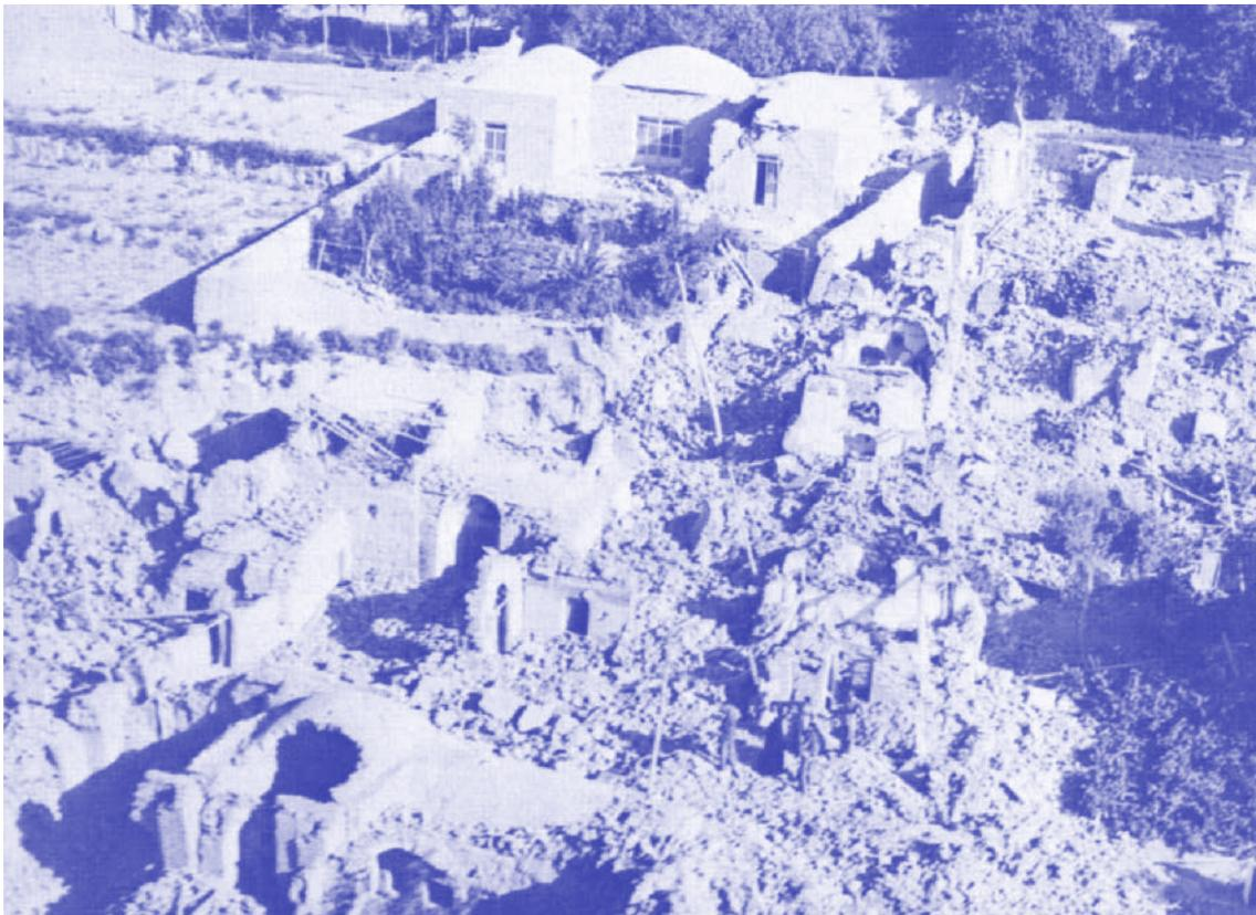
Housing with heavy roofs supported on unreinforced, dried mud (adobe) walls is one of the most vulnerable types of construction in seismic areas. This is indicated in an example of failure, with high loss of life, from an earthquake in Golbuf, Iran, in 1980.
